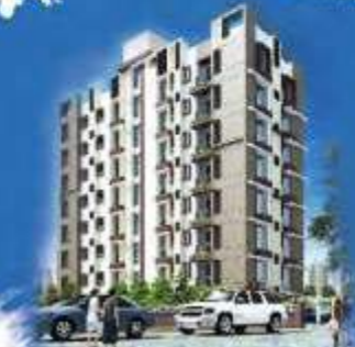
PRUDENT HABITAT Christopher Road, off EM Bypass
